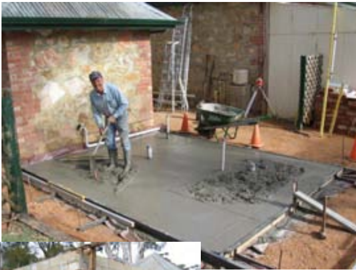
Progress with the new toilets. "Tiger" Hammerstein working on the concrete slab. Below: Work on the walls is very "fiddly" but the results are excellent thanks to "Shine" and Village volunteers (July 7th)
